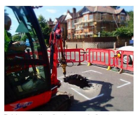
The hole was caused by a collapsed sewer more than five metres underground.
